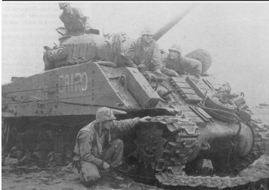
Waiting for Three-A? It was the job of a tank crew to make repairs and this tank has already backed off a tread broken by a mine. Now for the heavy lifting. The boards on the side of the tank are protection against magnetic "sticky" bombs.
