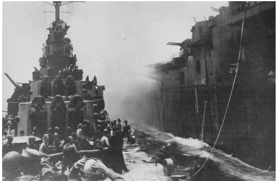
THE LIGHT CRUISER Birmingham rigs lines and fire hoses to the stricken light carrier Princeton and sends a party of firefighters on board at shortly after 1000. Princeton had been hit by a single 550-pound bomb that started internal fires. On the hangar deck, exploding torpedoes blew both fore and aft elevators out of their holes. Flames threatened both torpedo and gasoline stowage.
