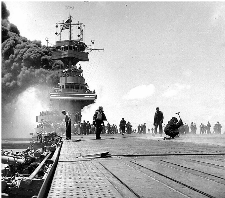
POUNDRING THE LUMPS OUT of Yorktown 's flight deck was only part of the effective damage control that enabled the ship to go from dead in the water to 20 knots and resume flight operations, but enemy torpedo planes would arrive in about an hour.
