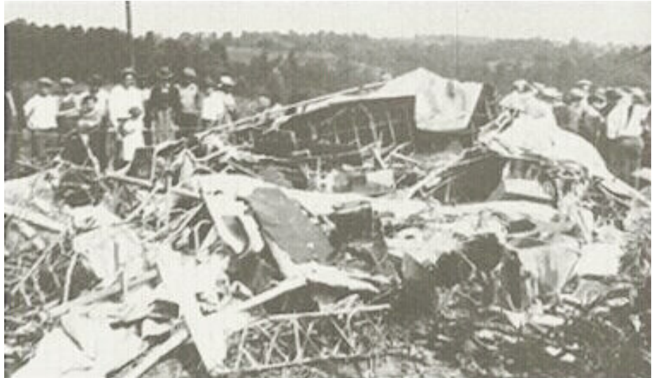
SIGHTSEERS GAPE at the wreckage of Shenandoah's center section. Four crewmen survived with injuries in this rubble, but four mechanics perished when their engine cabs broke free and plummeted to earth.
